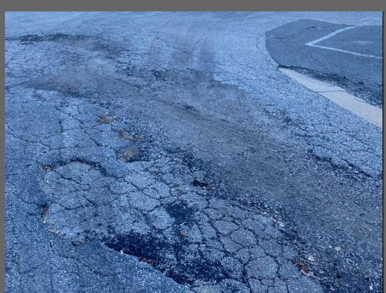
Images of damages at the site. The chimney (left) was struck by lighting and the vehicle lots (right) are riddled with large potholes.
