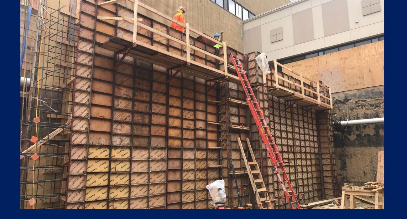
Pictured here is the setup before a concrete pour for one of the basement walls. It took many days to get the wall pour set up as we would have to make sure each section was secure enough to support the concrete.
