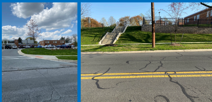
Both these images were captured at Sargent Shriver Elementary School in Silver Spring, MD by myself. The image on the left shows the cracked streets and uneven pavement right in the front entrance of the school, a low point for its infrastructure. The image on the right shows that the school is accessible by both able and disabled people.
