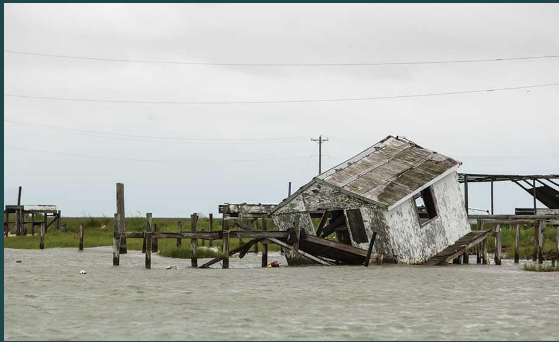
House on Tangier Island: This is a house on Tangier Island in the South Chesapeake Bay that has had its foundation eroded away causing it to collapse. This type of erosion has been increasing the past few decades due to climate change. https://www.enr.com/articles/42492-erosion-trumps-sea-level-rise-on-a-small-settlement-in-the-chesapeake-bay
