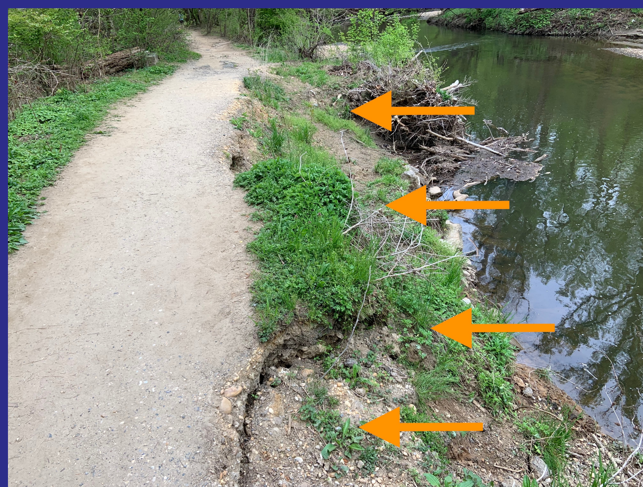
Fig. 2: Massive erosion present on a walkway, this presents a hazard to park goers especially at night where they may fall into the river at right
