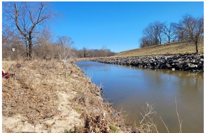
Figure 1: Channelized stretch of the Anacostia River with riprap placed on edges
