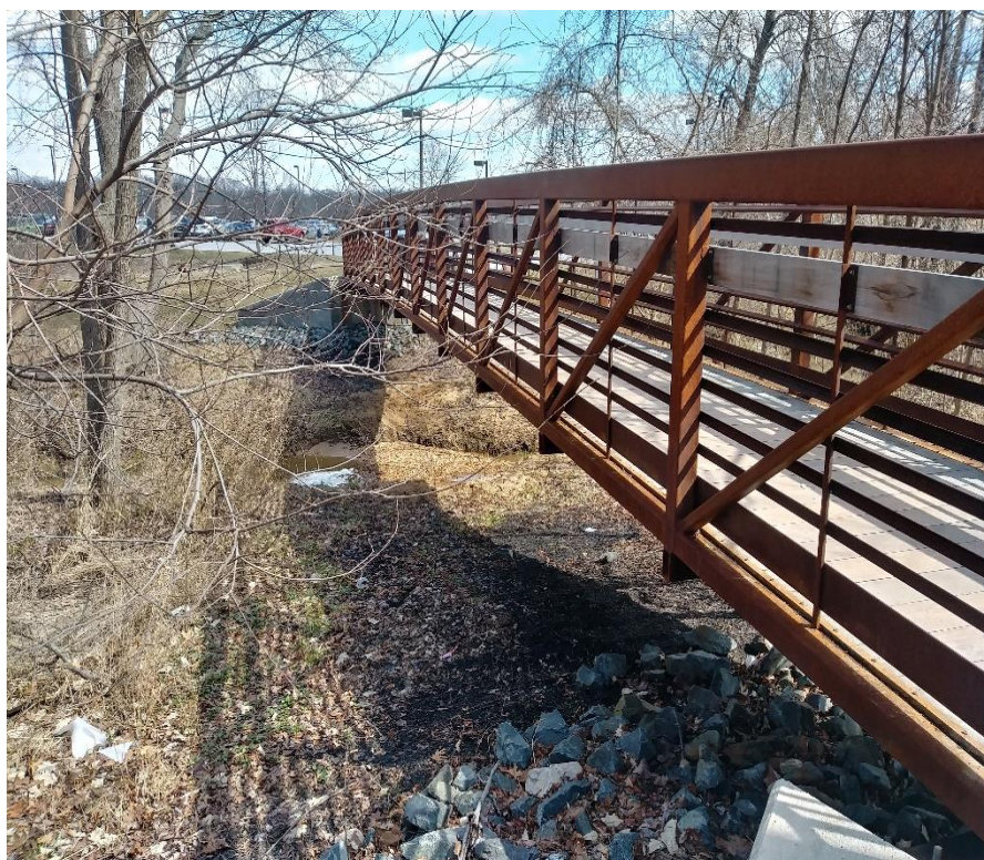
Figure 6: Site 7, taken during dry, base-flow conditions on 3/4/19.
