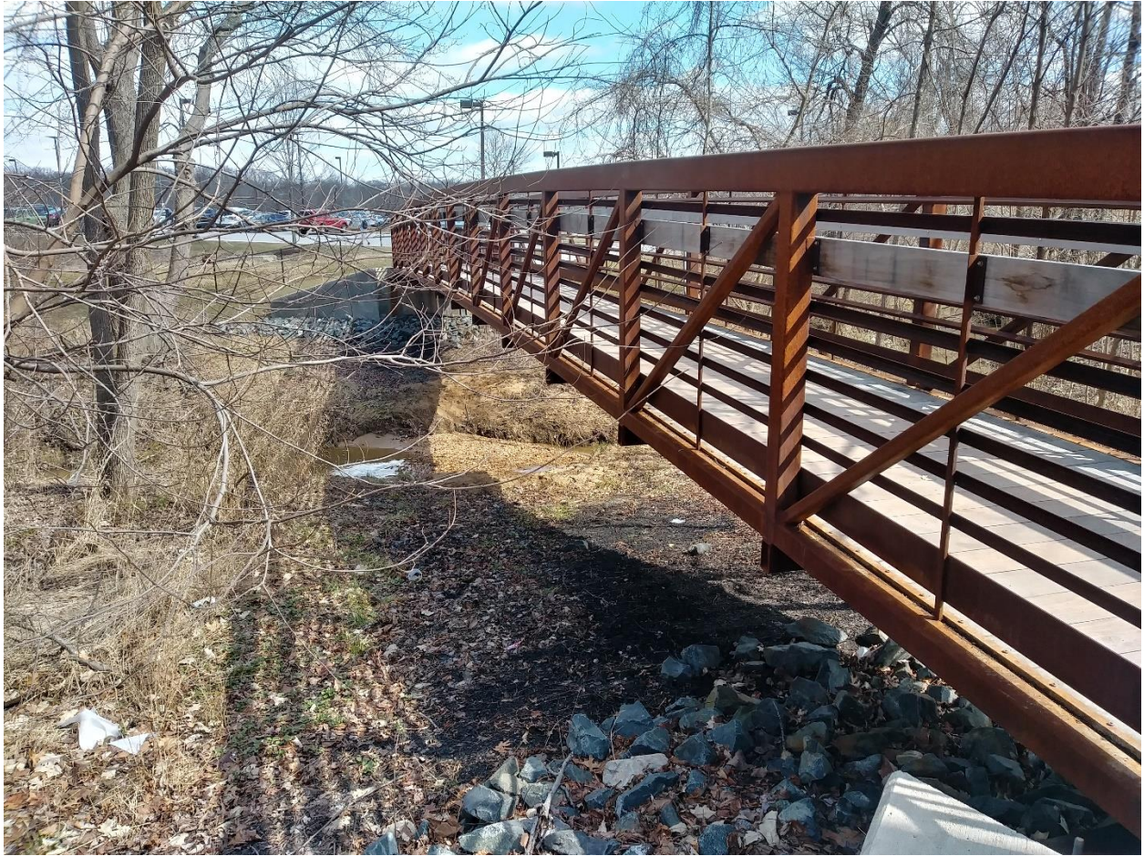
Site 7: 38°59'35.9"N 76°56'23.6"W. Water exits woods after flowing past wastewater outlets and buried sewer lines. Sampling is done downstream of bridge pictured, but upstream of Xfinity Center parking lot runoff input.
