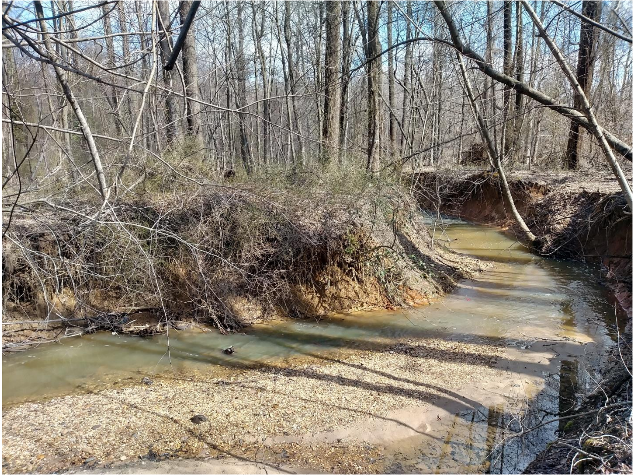
Site 5: 38°59'41.9"N 76°56'56.4"W. Water flows from site 4 past a pond, under and across the road coming out in another metal culvert. Flows N-NE parallel to the road for 350 ft through woods behind Oakland Hall.
