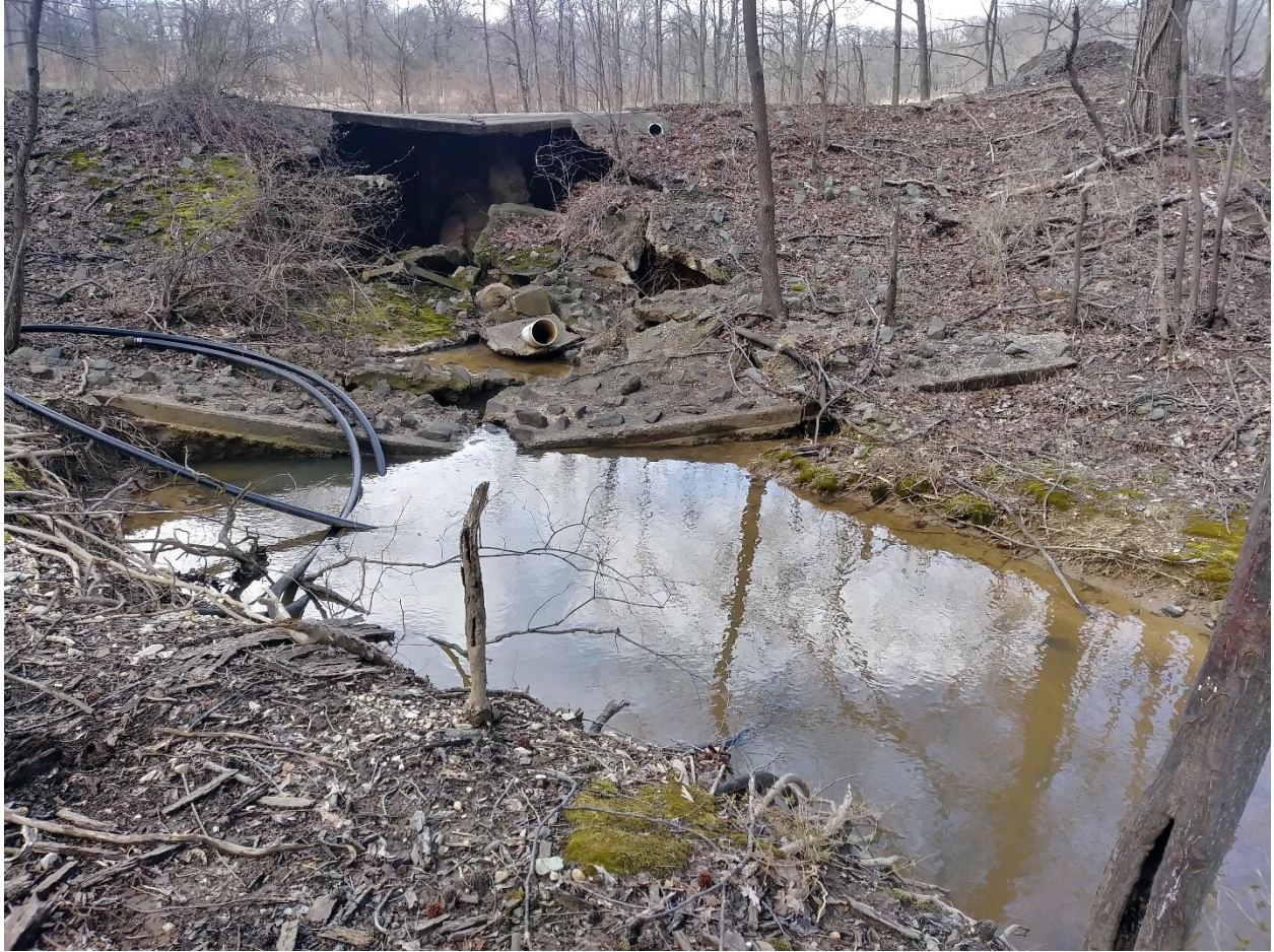
Site 3: 38°59'40.9"N 76°57'15.4"W. Outlet for water that flows through marsh. Water flows E-SE through woods to site 4.
