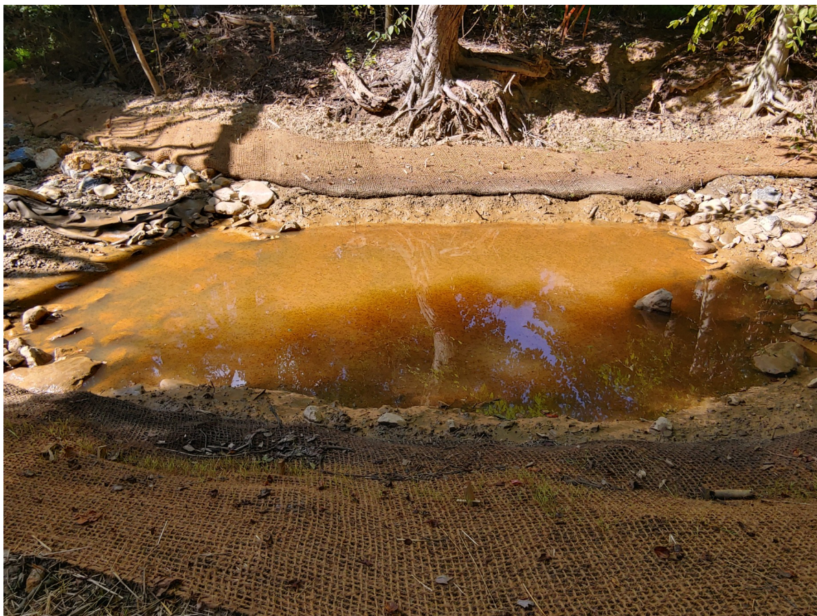
Fig. 2.2 One of the stormwater step-pools located along Campus Creek. This is one sampling area for the RSC site. The opaque, orange color is likely due to iron flocculation. Photo courtesy of Kelsey Wood, 2019.
